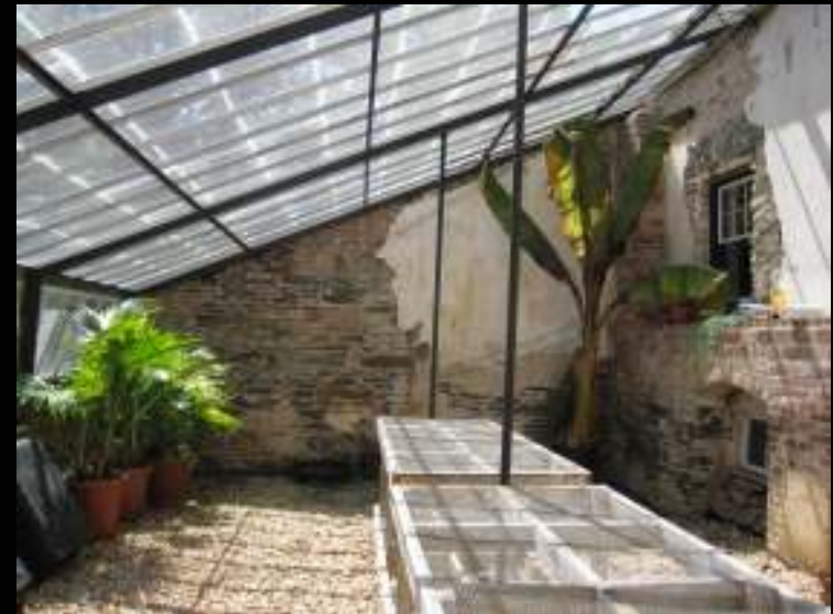
Oatlands Greenhouse, Built circa 1810 Phase 1 restoration 2001; Phase 2 will be 2011
